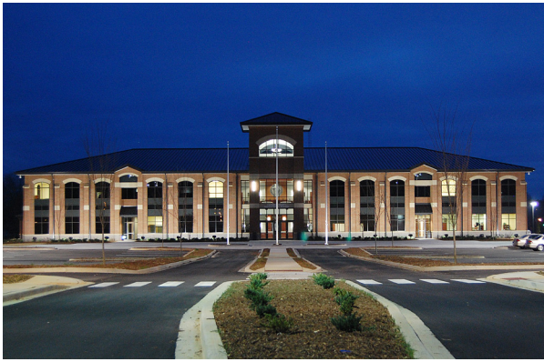
Administration building, Gaffney, South Carolina
